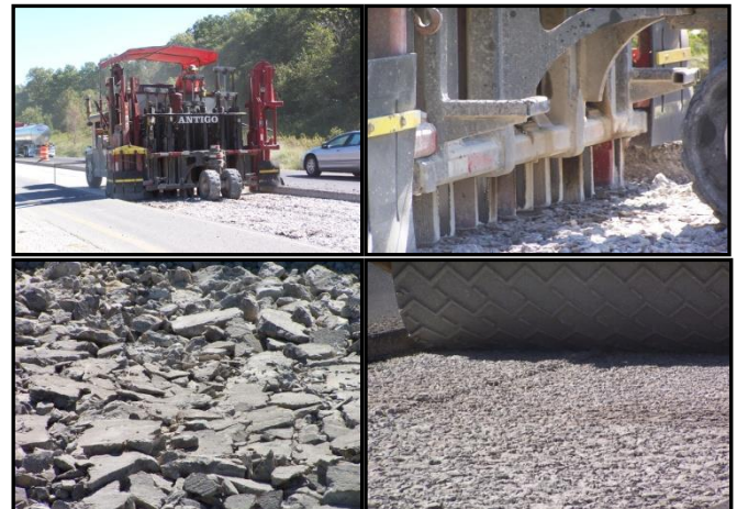
Rubblized In-place Concrete
