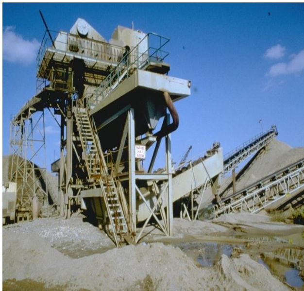
Sand &amp; gravel production plant
