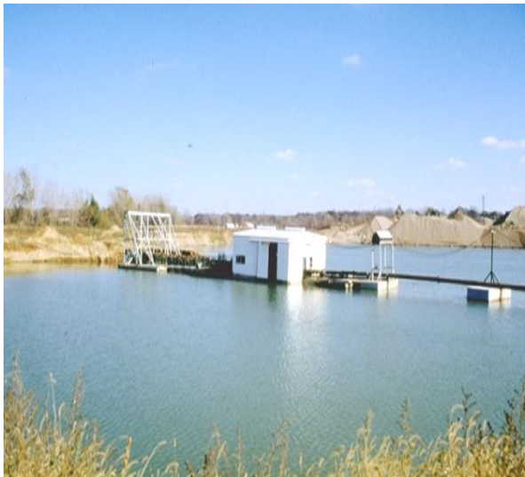
Sand and gravel pumping operation
