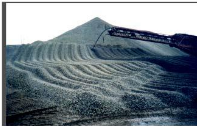
CREATING WINDROWS WITH A TELESCOPING CONVEYOR F23
